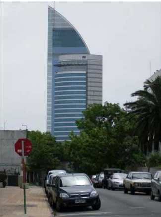
The ANTEL telecommunications Building
