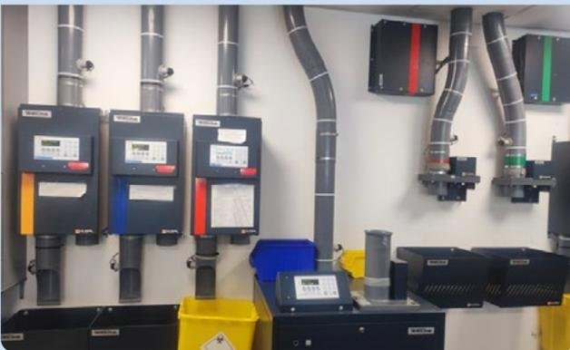
*The dispatching area of the lab with a pneumatic tube system*
